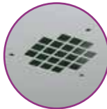
Orifices de ventilation
